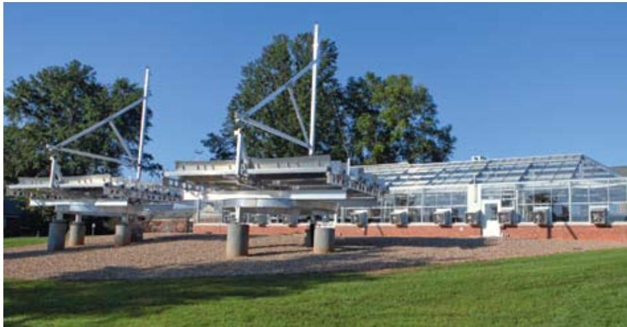
Of the Living Machine, Redderson says, “The wastewater reclaim system processes up to 5,000 gallons a day of sanitary sewer water. The reclaimed water, or graywater, can be pumped back into the building to flush urinals and toilets, which reduces our freshwater consumption by another 5,000 gallons a day. This is enough water to fill up the main campus fountain every four months, or enough water for 100 showers each day.”
